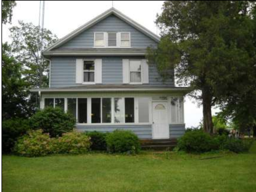
Clear Creek House, McNabb, Illinois Photo taken by Pam Timme
